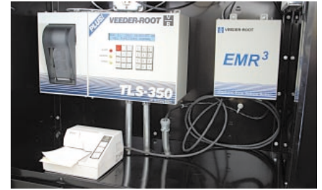
The EMR3 can be connected to any Veeder-Root TLS series automatic tank gauge for enhanced fuel monitoring capabilities.
